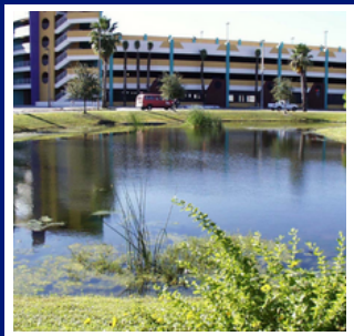
Retention Basin near a parking garage; source: Southwest Florida, WMD, 2005
